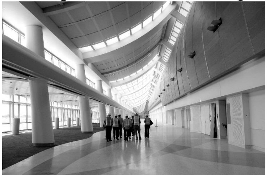
Cathedral-like North Concourse is almost finished at SJC – Northern Wings Photo
